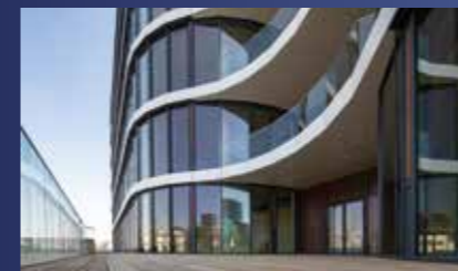
Kotelna Park II Prague, Czech Republic BREEAM "Very good" certified
